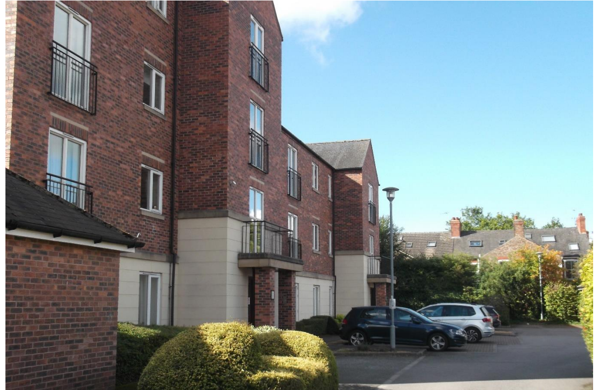
Neighbouring Building – Curlew House
